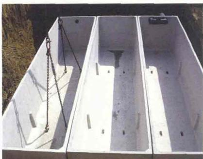
*Pircher is the name for state-of-the-art rolling systems designed to prevent overflows. Made with concrete tanks, they allow water to be preliminarily stored and let into the end receivers, as requested by authorities. These systems make it possible to set a standard water flow to the outlet and carry excess water – through a flow distributor – into the Pircher tanks, where it is stored and, at the end of the peak*
